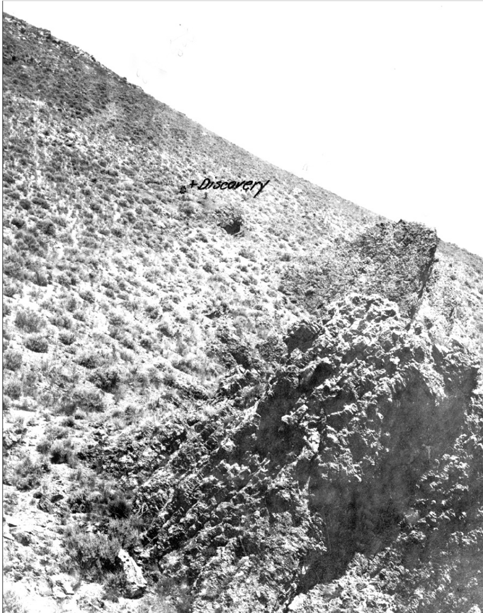
Figure 18. Discovery tunnel of the Nashville Lode Mining Claim, 1911. Photo from the patent case files, General Land Office, National Archives and Records Service, Washington, D. C.
