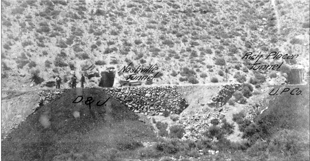
Figure 19. Union Phosphate Company's tunnel on the right (Rich Placer Claim) and the Nashville Lode Mining Claim tunnel on the left, 1911. Photo from the patent case files, General Land Office, National Archives and Records Service, Washington, D. C.
