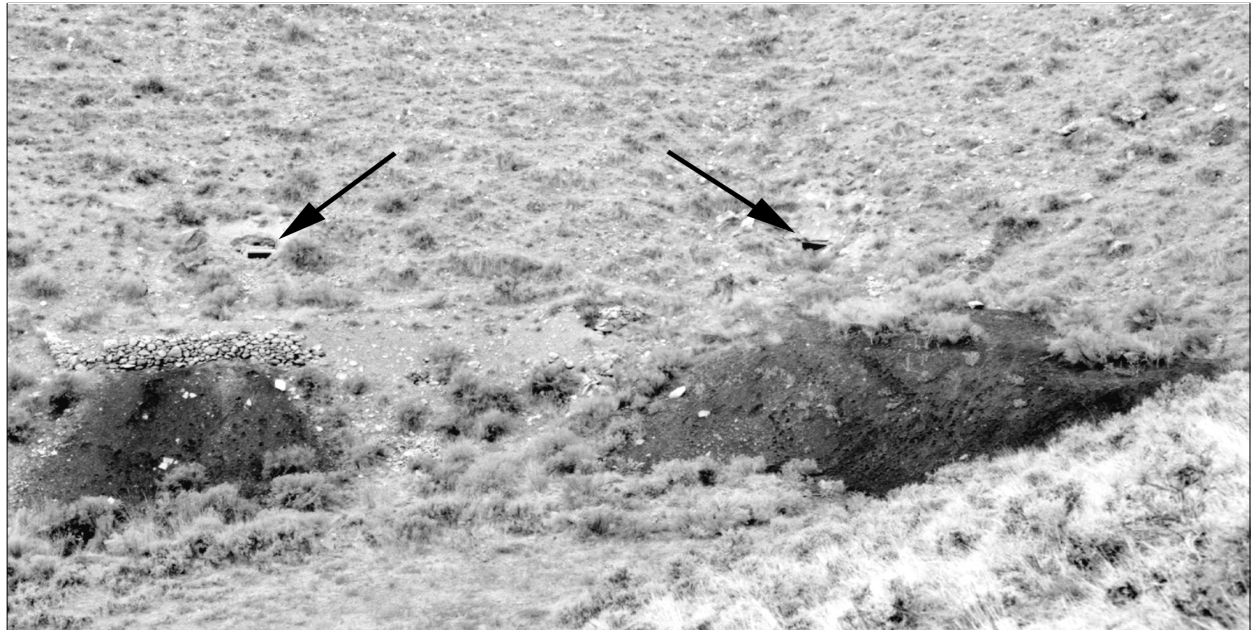
Figure 20. Union Phosphate Company's tunnel on the right (Rich Placer Claim) and the Nashville Lode Mining Claim tunnel on the left, September 9, 1996. Photo by the author.
